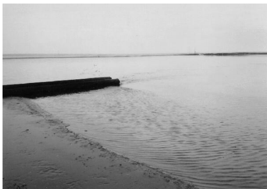
Fig. 1. Discharging pipes of produced water into surface pit at an oilfield
