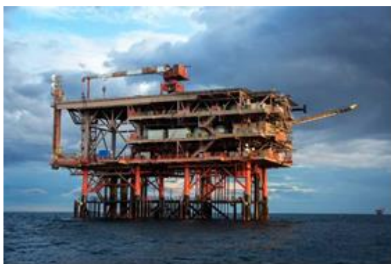
Figure 1. Rospo Mare B platform.
